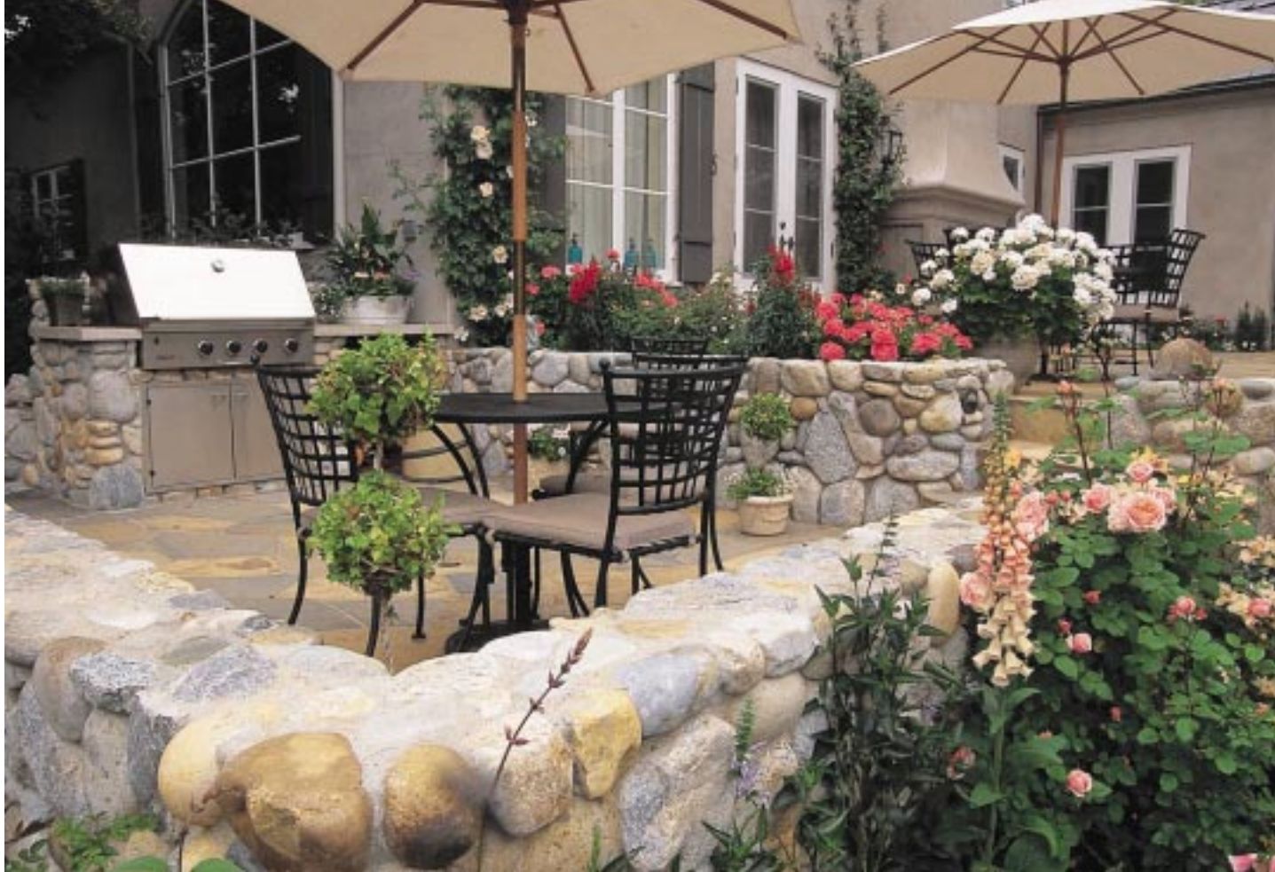
ABOVE: An 18-inch-high river rock wall encloses and surrounds the lower dining patio. Because Cynthia designed it at the height of a comfortable chair, the wall is ideal for extra seating during large parties.
